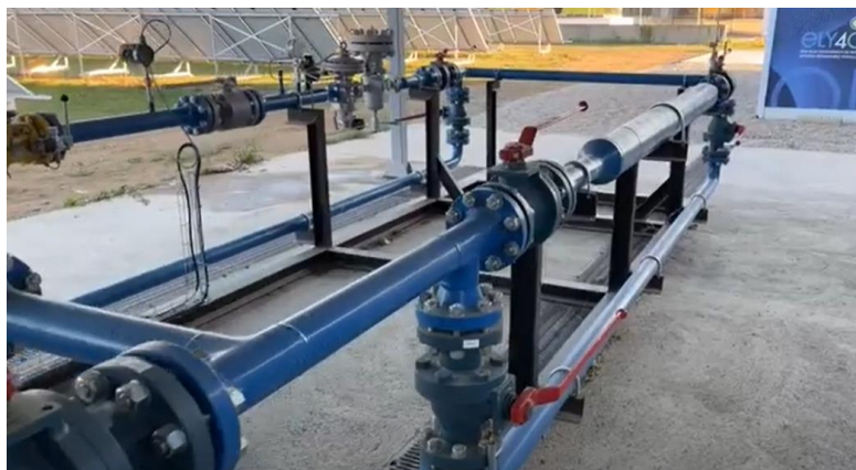
Figure 8. Welded pipe sections of the API 5L steel pipes
