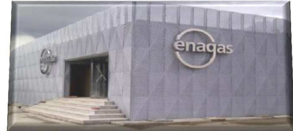
Zaragoza (DPC) Data Processing Centre
